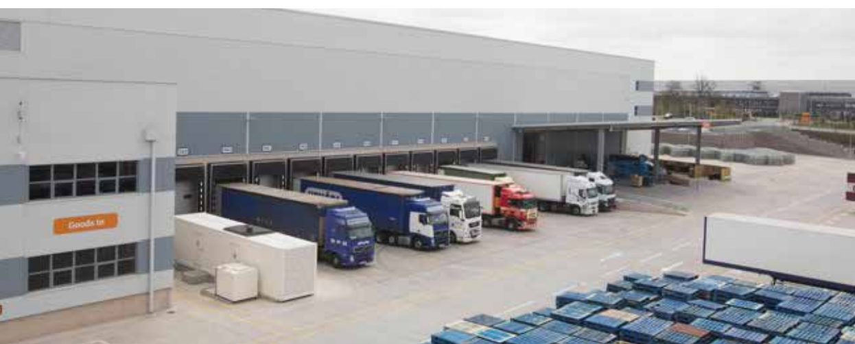
Daventry International Rail Freight Terminal. Developed by Sainsbury's and DHL.
